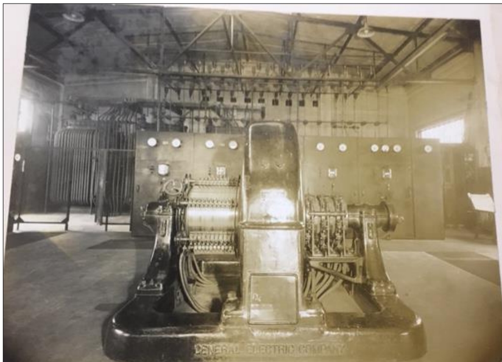
Figure 3: Interior of the #10 Substation looking at the south wall. 11 kV circuit breakers are in the background; overhead bus work; 2.3 kV circuit breakers are along the east wall (left); main 11 kV / 2.3 kV transformers are on the left. The rotary converter in the foreground supplies DC for underground haulage.
