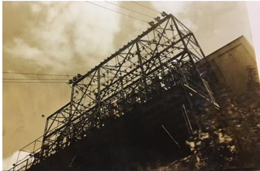
Figure 2: Exterior of the Hauto Navigation Substation looking south. Two incoming overhead feeders from the Hauto Power Plant are on either end. The Hauto Power Plant was to the north of this building.
